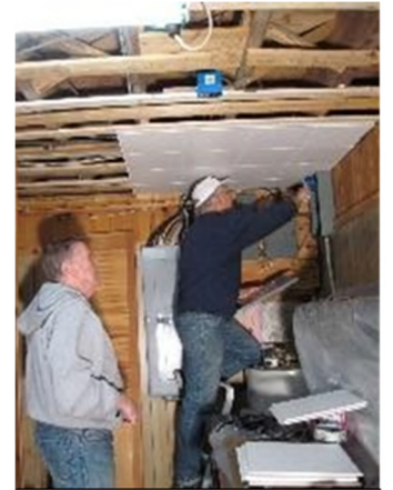
Pat and Bert putting up ceiling in kitchen at church
